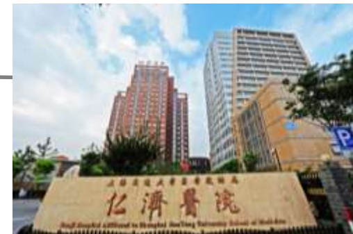
East Campus Headquarter
